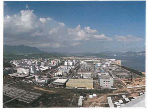
Tai Po Industrial Estate
